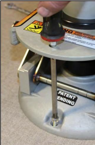
*Figure 16: Turn Screws into Floor*
