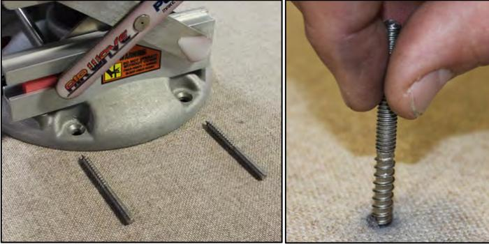
*Figure 9: Insert Hanger Bolts*
