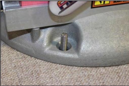
*Figure 11: Place AirWave™ Pedestal over Hanger Bolts*
