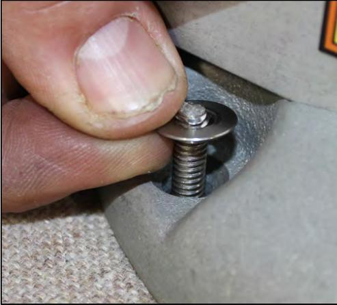
*Figure 13: Place Tapered Washers over Hanger Bolts*
